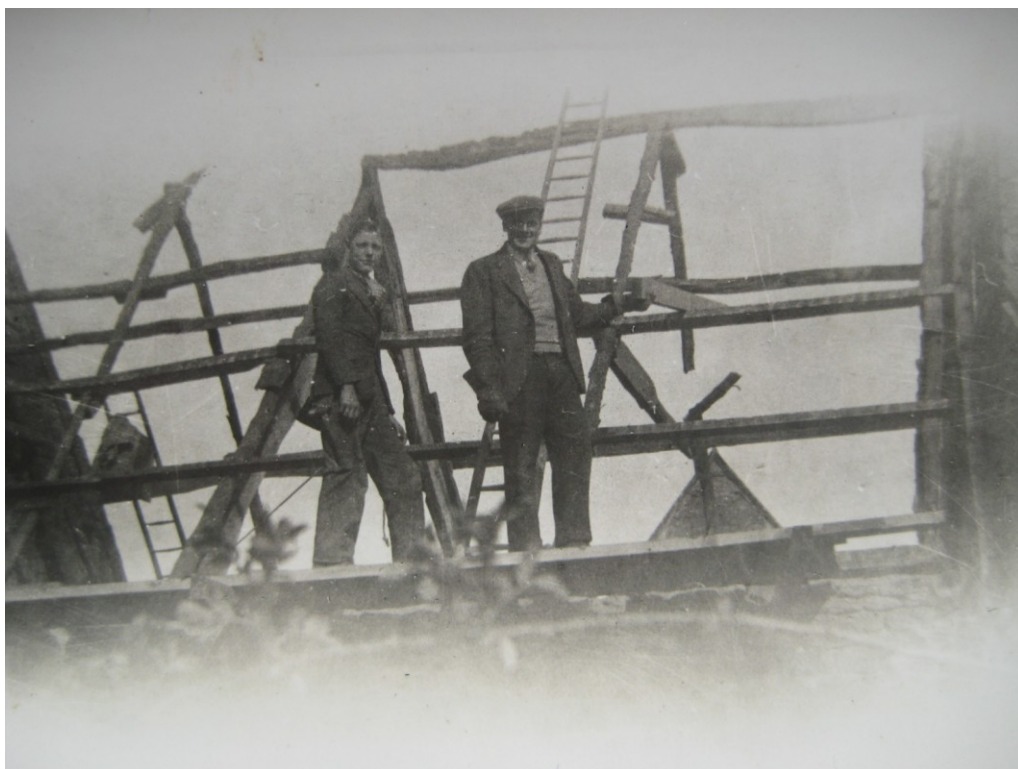
The roof of the cross-wing, after stripping of thatch
