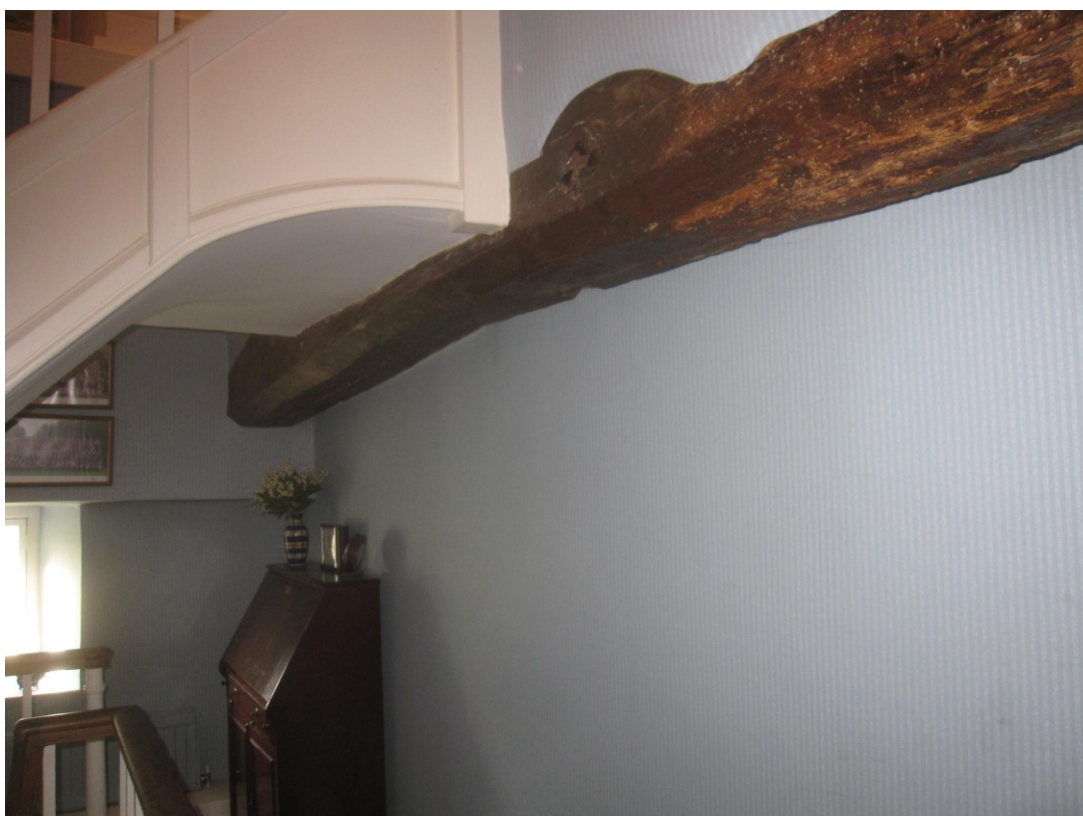
The first floor beam spanning west-east to the cross-wing
